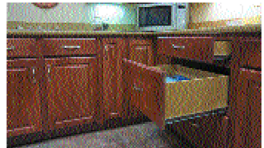
Provide full extension drawers on all lower cabinets instead of doors and fixed shelving, affords full easy access and minimized back strain and injuries. Install easy-to-grasp drawer and door handles or knobs.
