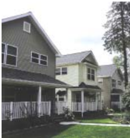
Local community development and planning officials need to take a fresh look at manufactured housing, such as the Noji Gardens project in Seattle, Wash.
